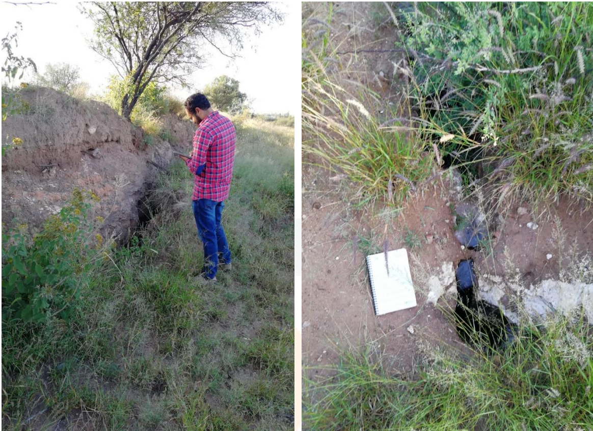
Figures 3a and 3b. Surficial view of the Oriente fault located in a vast non-urban area inside Aguascalientes city. The large number of fractures associated to the master fault has impeded the construction of more infrastructure at this locality.
